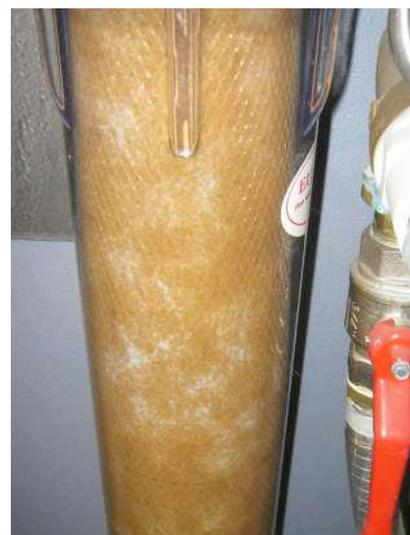
Figure 3: Red-brown pre-filters are certain indicators for damage caused by corrosion contamination.
